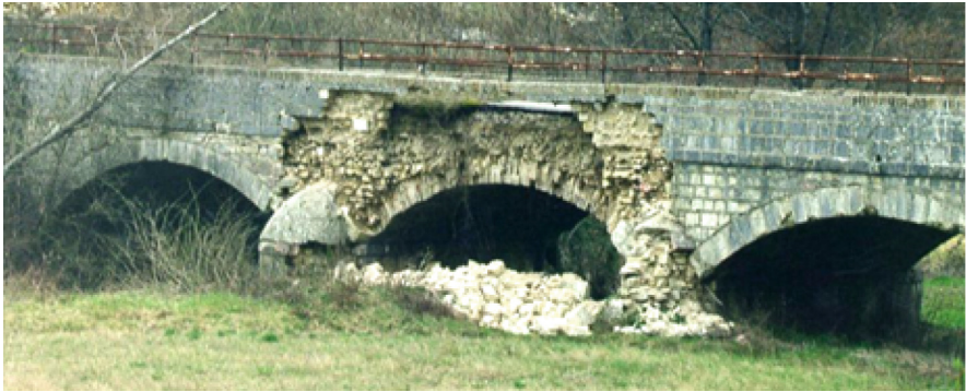
Fig. 12. Seismic damage to a road bridge in Preci (IT) 1997 earthquake (L. Gambarotta).
