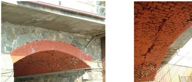
Fig. 28. Longitudinal cracks below the spandrel to overloading of the spandrels
