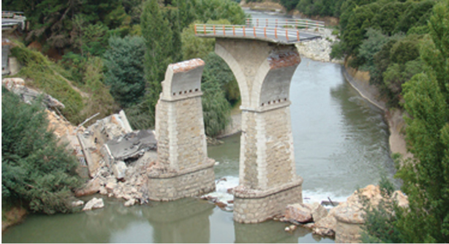
Fig. 13. Collapse of a masonry bridge on the Claro river (Chile) due to longitudinal seismic action, 27 th of February 2010.
