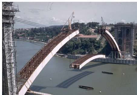
Fig. 35. Completion of the falsework for the execution of the first of the twin arches [19] JAE and IP
