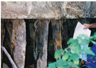
Fig. 10. Partial collapse due to wooden pile rot [2] a2p archive
