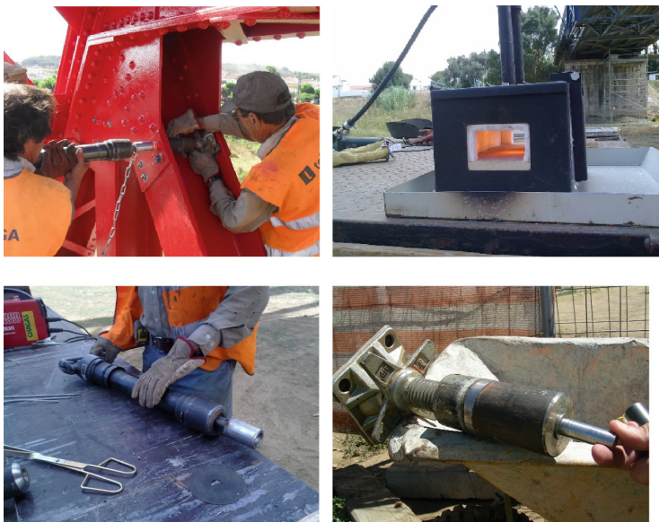
Fig. 20. Application of rivets in rehabilitation works a2p archive
