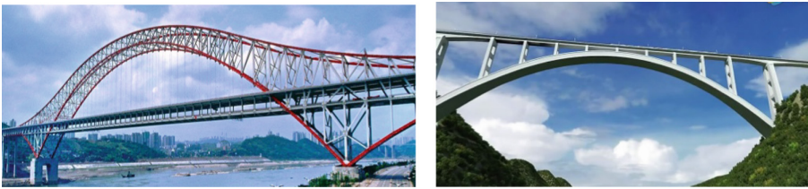
Fig. 10. Chaotianmen (steel-552 m) and Qinglong railway bridge (concrete-445 m)
