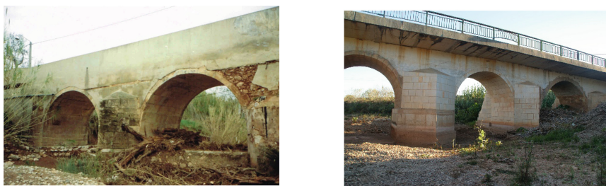
Fig. 8. Deck widening with precast slabs longitudinal posttensioned [2] a2p archive
