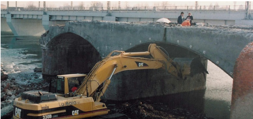
Fig. 9. Multi-span railway bridge on the Tanaro, Alessandria (IT) during demolition.
