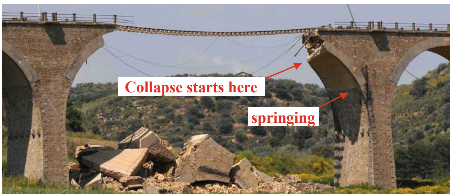
Fig. 7. Collapse of a span of a railway multi-span bridge
