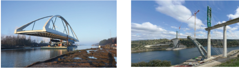
Fig. 7. Construction methods for arch bridges
