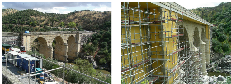
Fig. 7. Deck widening with a new prestressed concrete slab over the masonry bridge, [2] a2p archive
