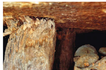
Fig. 10. Partial collapse due to wooden pile rot [2] a2p archive
