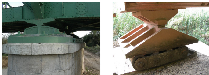
Fig. 21. Steel Fixed and sliding bearings a2p archive
