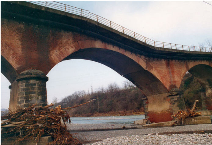
Fig. 29. Excavation of a pier - 2002. Note that the base of the pier had been “protected by means of a symmetrical r.c. collar. Bridge on the Scrivia river, District Road 141 – Val Borbera – IT
