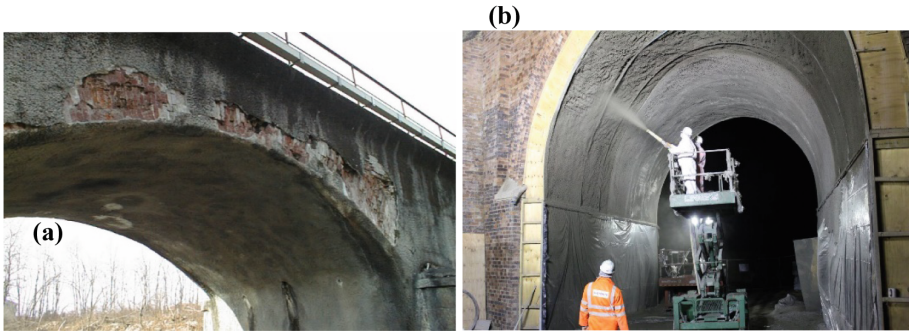
Fig. 24. Shotcreting of a masonry bridge (a) extended to the spandrels; (b) limited to the arch.
