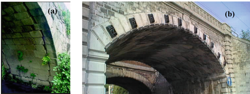
Fig. 25. Transversal tie bars from one side of the arch to the opposite side (a) detachment of the spandrel from the arch barrel and (b) Massarenti Bridge , Bologna (courtesy RFI).
