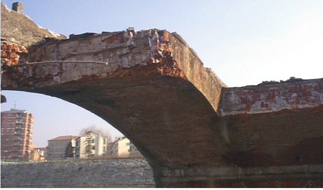
Fig. 10. Bridge of Fig. 9: the arch consisted of 3 parallel arches connected by transversal ties.
