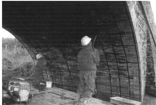
Fig. 23. Connection of stainless steel bars to the arch barrel [36]
